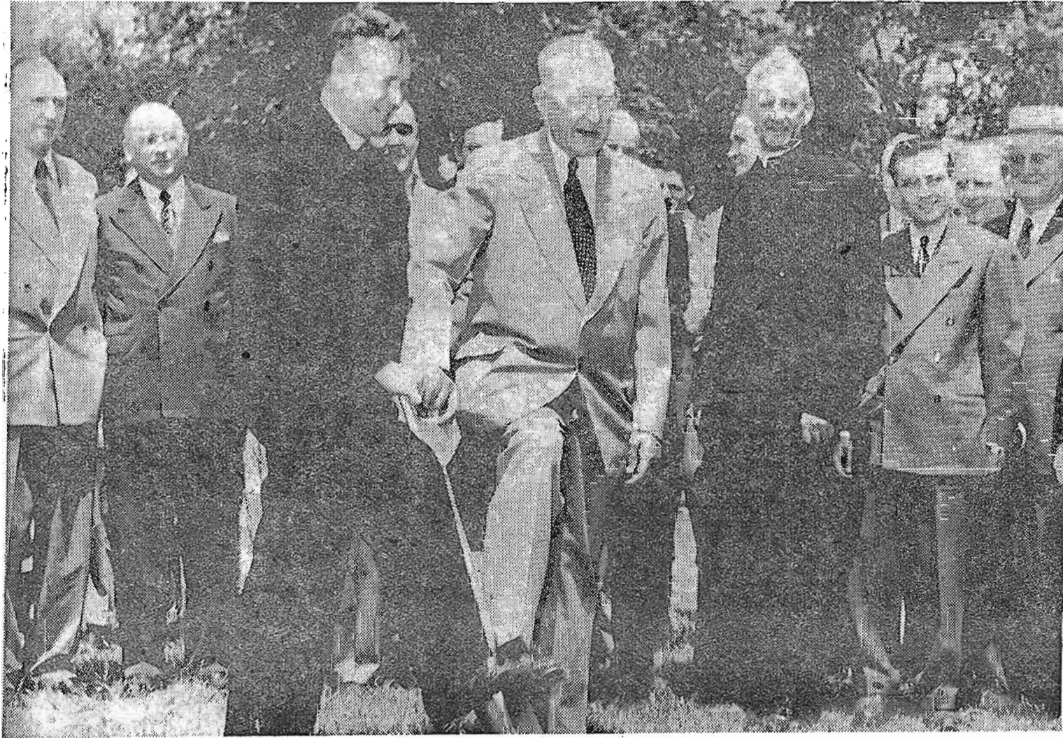
SPADEWORK: The Very Rev. William J. Millor S.J., former University president, helps to break ground for the library. This scene which took place in May of 1949 paved the way for the erection of the now-completed library which was formally dedicated this afternoon. The building took only a little over one year to complete to such an extent that it was available for student use. Among the features included in the library besides the books are class rooms, map rooms, and the theater. The library was completed at a cost of over one million dollars.
