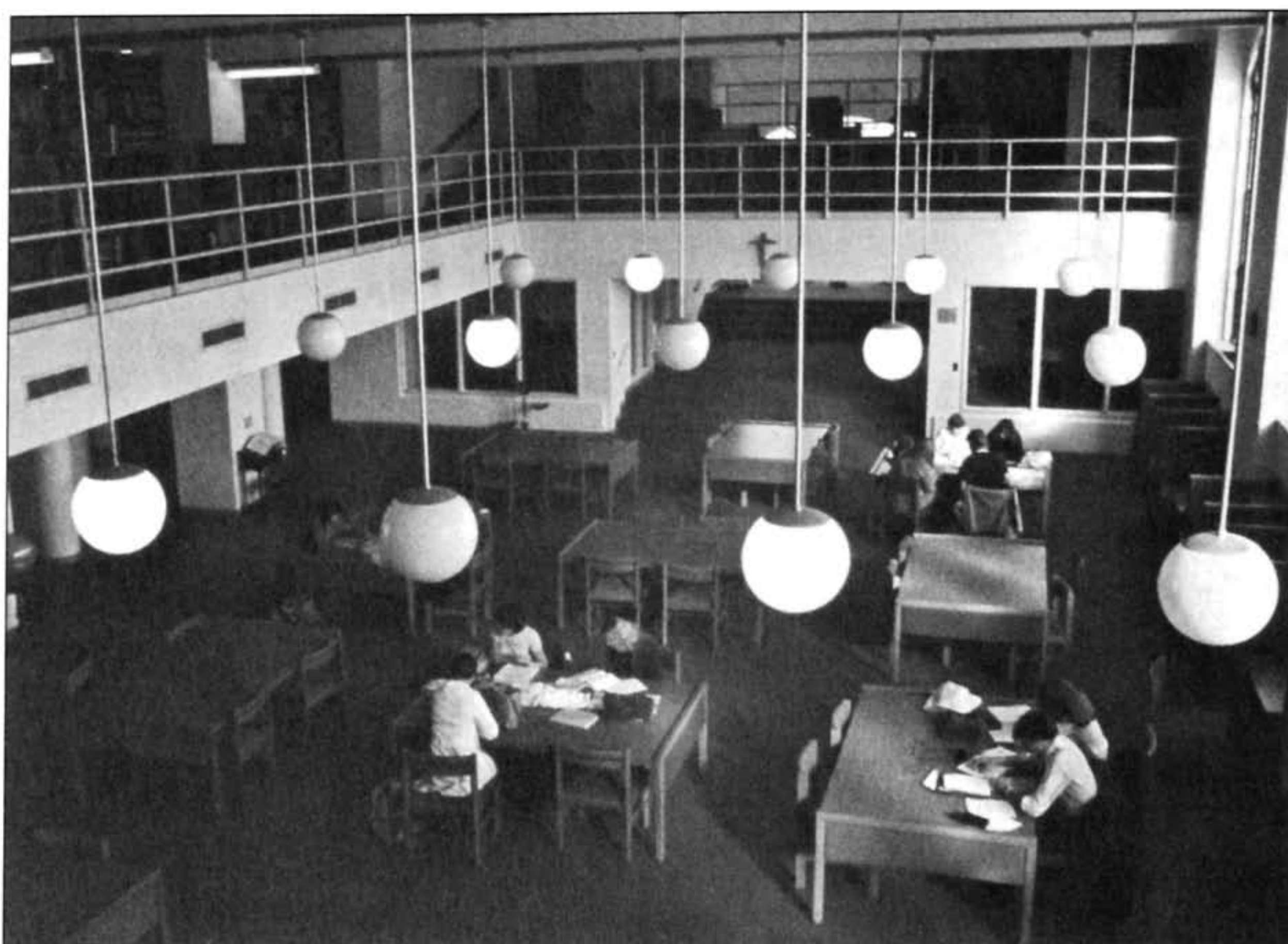
The first floor of the new Library, 1980.
