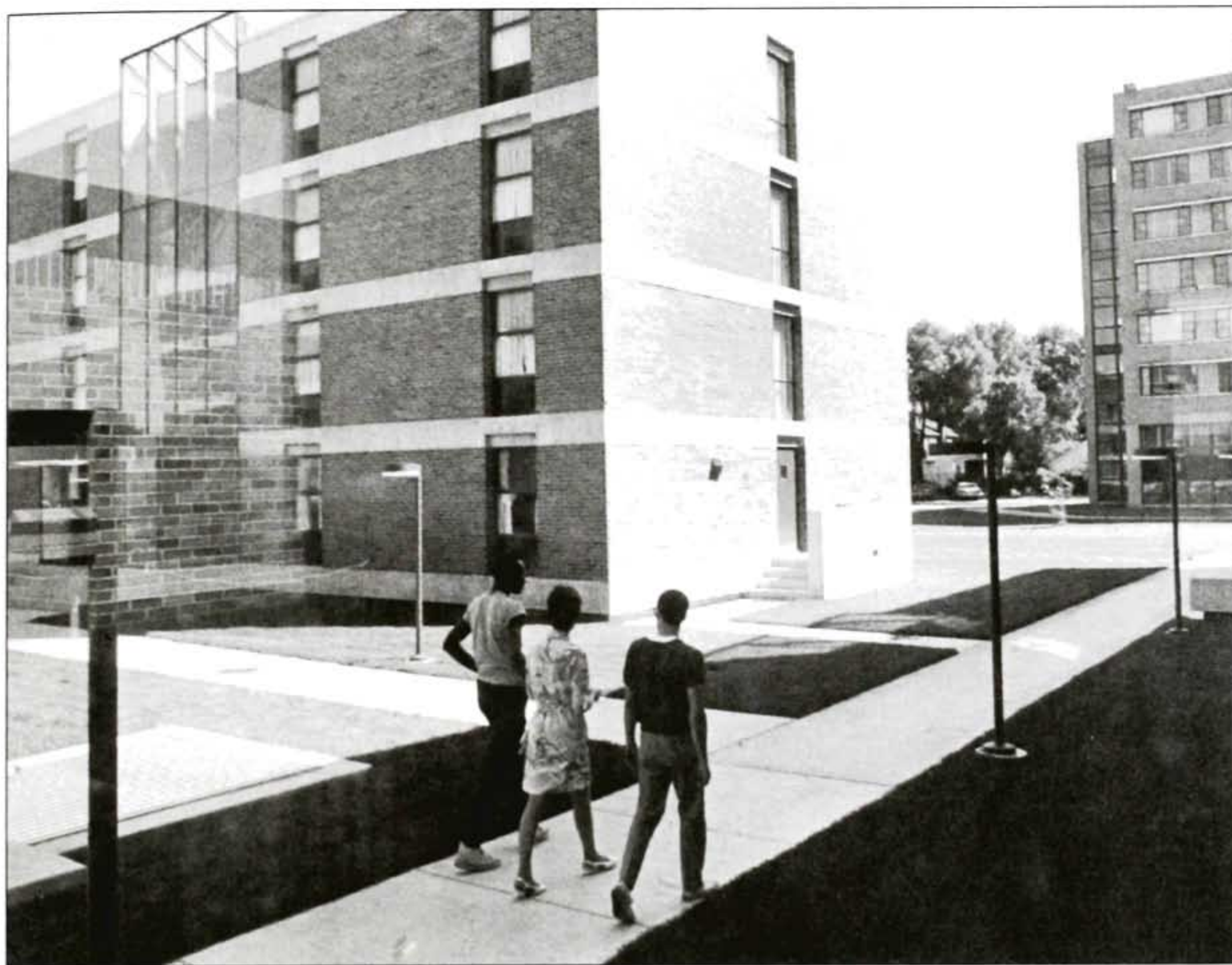
A new dormitory complex, the Quadrangle or "Quads," was opened in fall 1969.
