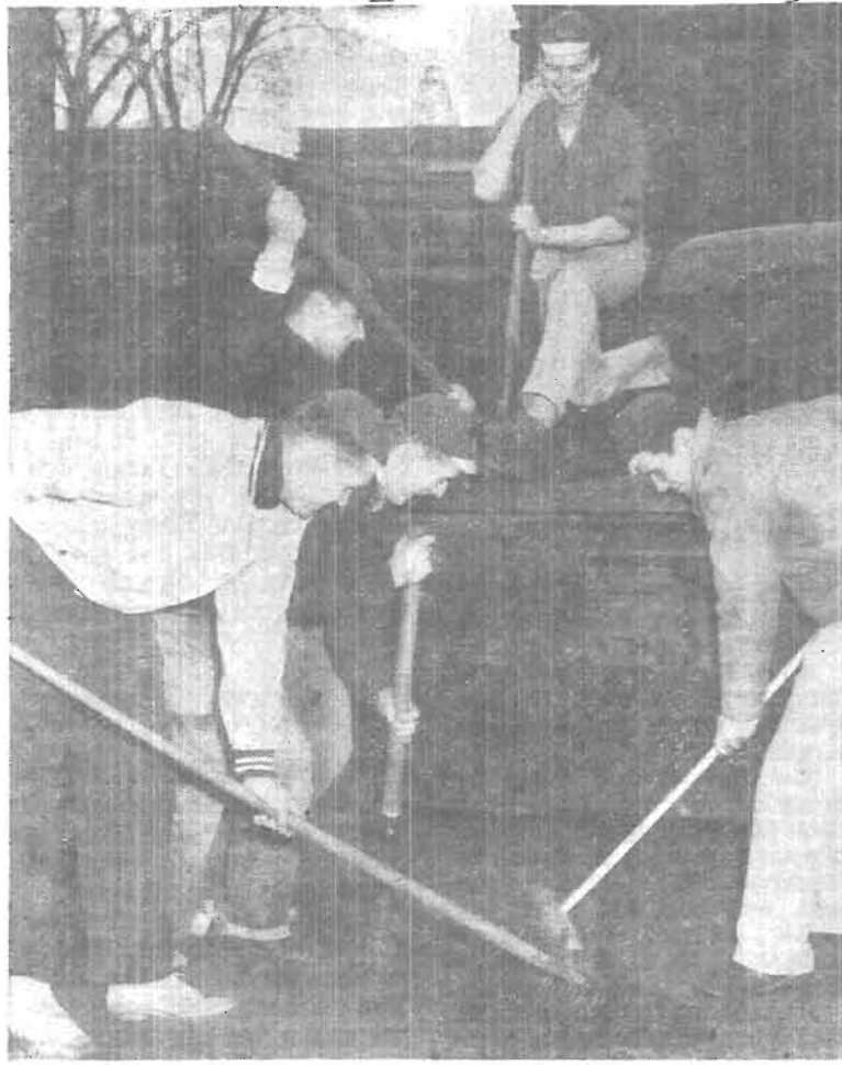
Pledges of Kappa Sigma Kappa improve the campus by shoveling cold-pack from truck to chuck holes in University roads.
